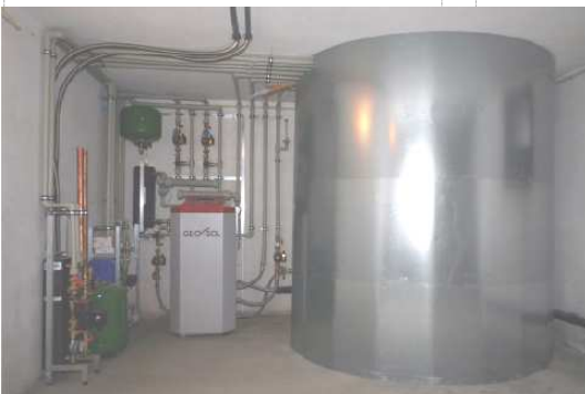
Picture 5: Heat pump and storage tank [source: GIWOG]
