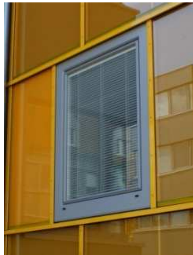
Picture 4: Façade integrated window at Dieselweg No.4 [source: AEE INTEC]
