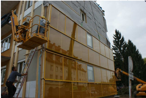
Picture 7: Mounting procedure of the modules [source: AEE INTEC]
