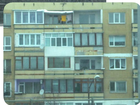
Multifamily building in Sofia. One building can have as many types of windows as there are apartments.
