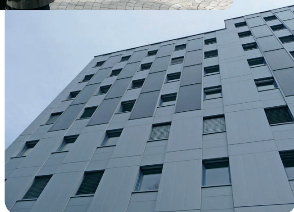
The Friedrich Stiller homes for students. The TRECO group and SQUARE group in front of the building. Façade with integrated solar collectors.
