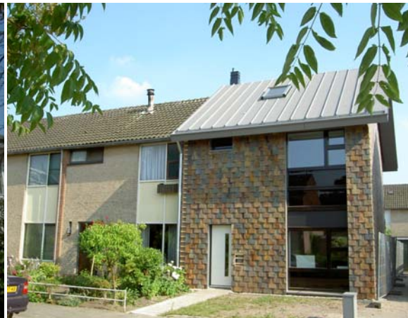
Figure 57 Test house with timber frame elements with cellulose insulation and prefabricated timber roof.
