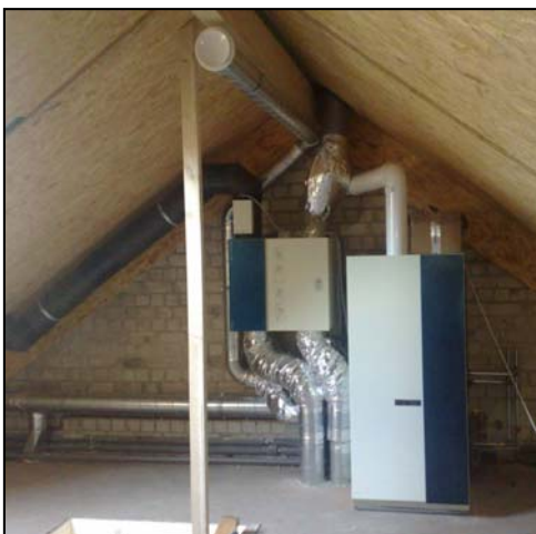
Figure 55 New compact heat and ventilation system.
