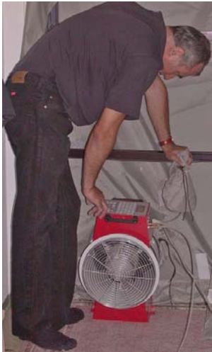
Figure 42 Testing the air tightness of a wall during the construction stage in order to verify air tightness. (Source: AEE INTEC)
