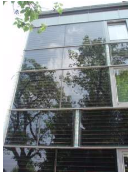
Figure 20 Solar thermal façade collectors at Dieselweg, Graz. (Source: AEE INTEC)
