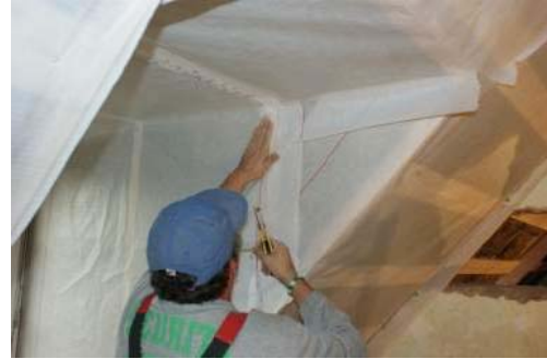
Figure 10 Making the attic airtight at Dieselweg, Graz. (Source: AEE INTEC)
