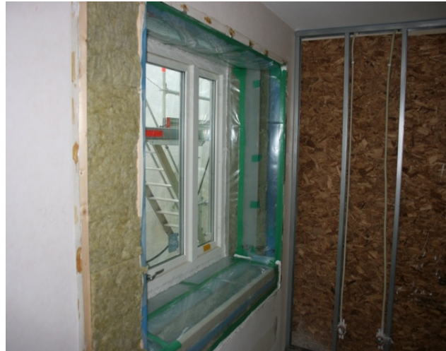
Figure 43 An example of an air tight solution of a window opening. (Source: SP)
