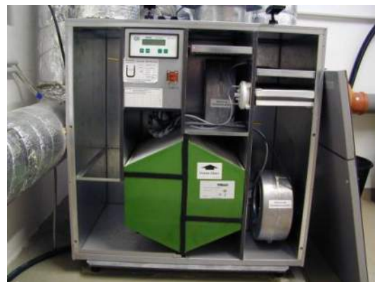
Figure 24 Ventilation device with integrated heat recovery. (Source: AEE INTEC)
