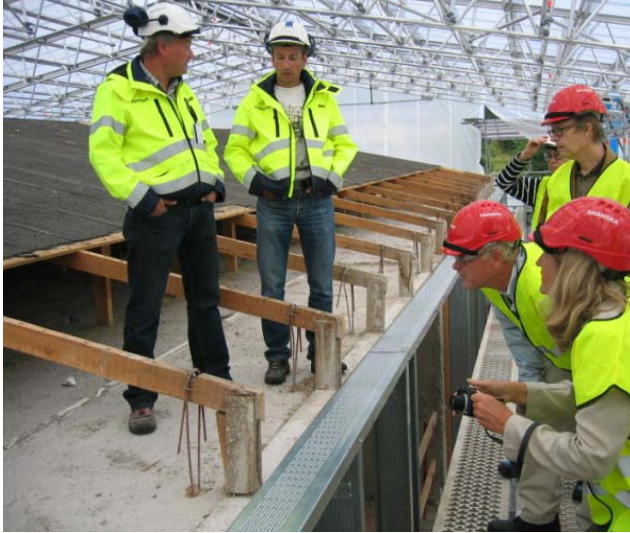
Figure 40 Moisture rounds at the building site. (Source: SP)
