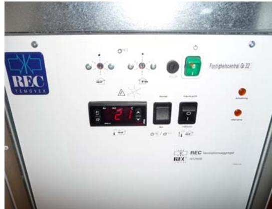
Figure 22 Display for the apartments ventilation units with heat exchanger. (Source: SP)
