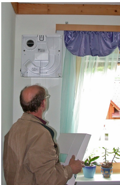
Figure 45 Installations check-up during inspection rounds. (Source: AEE INTEC)
