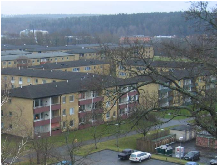
Figure 2 Multifamily housing complex in Brogården built 1963-1973, Alingsås, Sweden.
