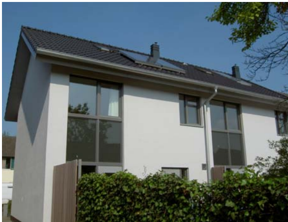
Figure 56 Test house with external EPS insulation and plaster and prefabricated timber roof.
