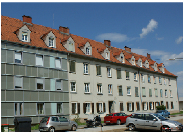
Figure 50 The last part of the long building row is owned by different owners. They did not want to join the renovation – so their building remained as before. Even the space heating is like it was before; everybody has to care for himself/herself (Source: AEE INTEC).
