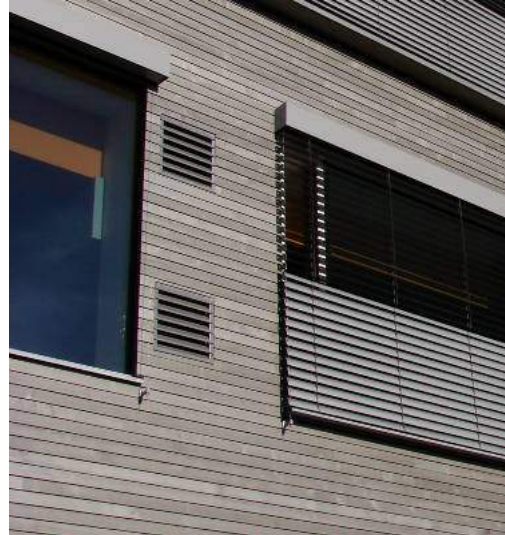
Figure 12 External solar shading reduces cooling demand. (Source: AEE INTEC)
