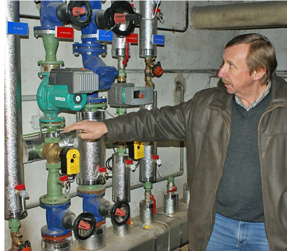
Figure 29 Inventory of installations (Source: AEE INTEC).
