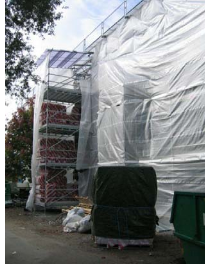
Figure 41 Weather protection to keep the building site dry. (Source: SP)
