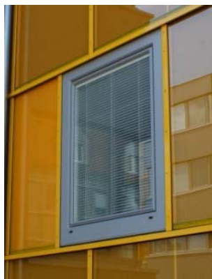
Figure A5: Pre-fabricated façade module with integrated window [source: AEE INTEC]
