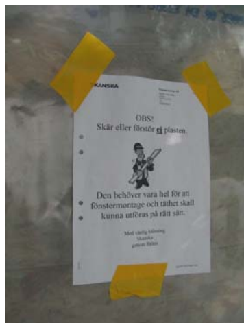
Figure 21 The workers were reminded of the importance of the air tight layer everywhere.
