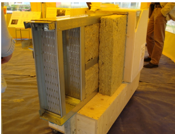
Figure 20 A prototype of the light in-filled walls was built before building at large scale.
