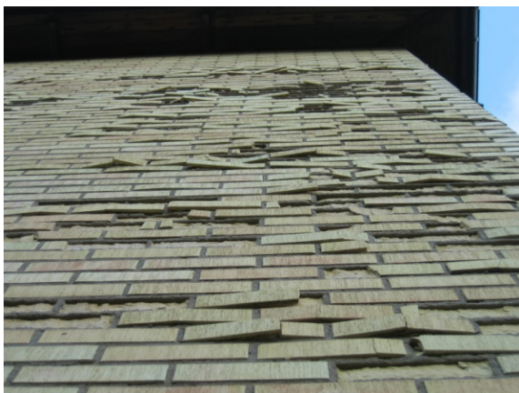
Figure 6 The brick façade was damaged by frost and had to be torn down.
