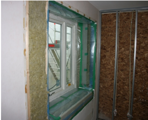
Figure 22 An example of an air tight solution of a window opening.
