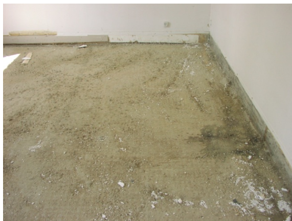
Figure 7 The ground slab had moisture damages that had to be taken care of.
