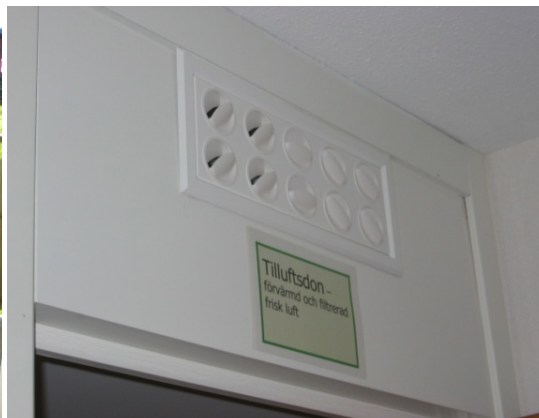
Figure 19 The sign explains that this is the supply air duct for pre heated and filtrated, fresh air.
