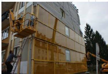
Figure A10: Mounting procedure
