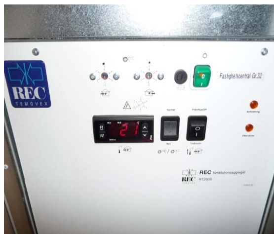
Figure 38 Air treatment system unit for a single apartment, used in building D.
