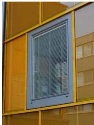
Figure A5: Pre-fabricated façade module with integrated window [source: AEE INTEC]
