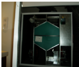
Picture: Open individual ventilation and heat recovery equipment
