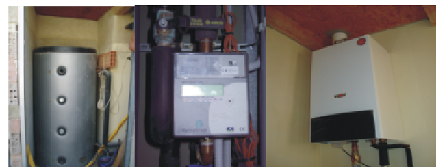
Picture: Hot water tank, thermal energy meter, condensation boiler
