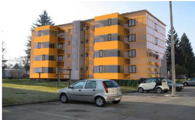
Figure 4: View on renovated building [source: GIWOG]
